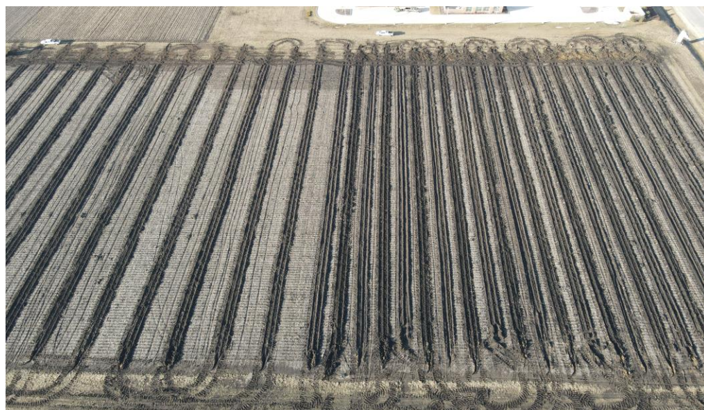
Figure 2. 15' and 30' Pattern Tile Installation
