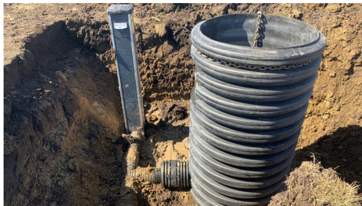
Figure 3. Gate Structures to Control Water Table
