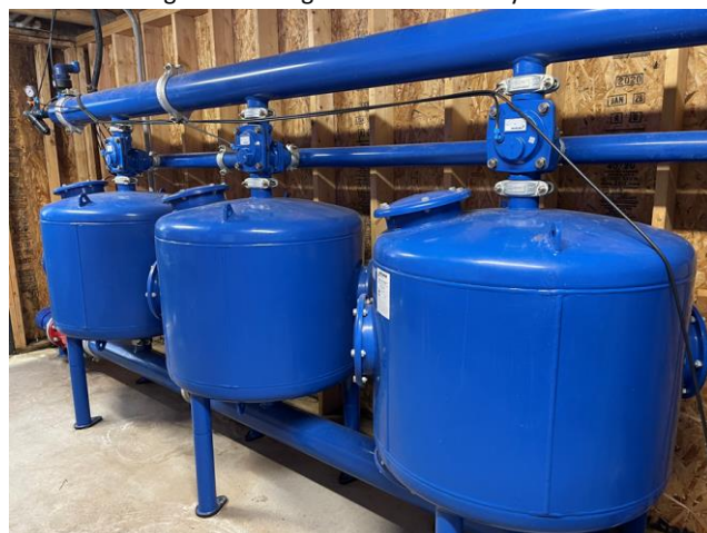
Figure 9. 3-Stage Sand Filtration System
