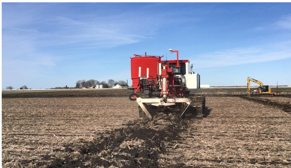
Figure 2. 15' and 30' Pattern Tile Installation
