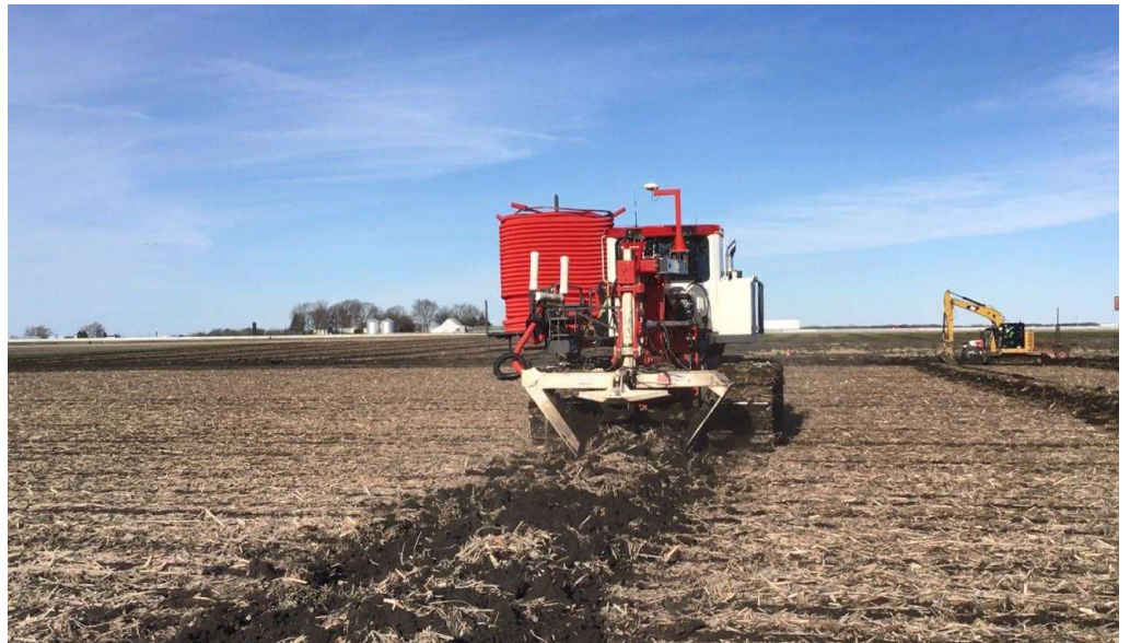
Figure 1. Tile Installation
