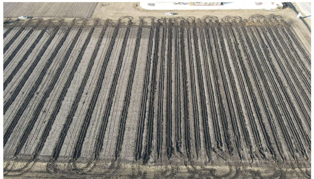
Figure 2. 15' and 30' Pattern Tile Installation
