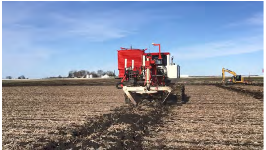
Figure 4. ADI V-Plow Tile Installation
